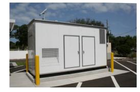
• Structural concrete precast wall panels and double "T" precast concrete roof system
