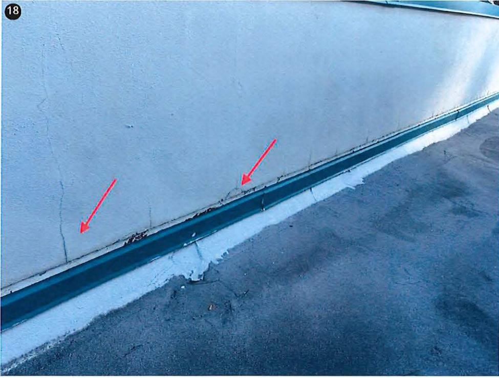
As the stucco continues to absorb water, particularly in this area, it can allow water into the building. Stucco repairs will be needed throughout the building.
