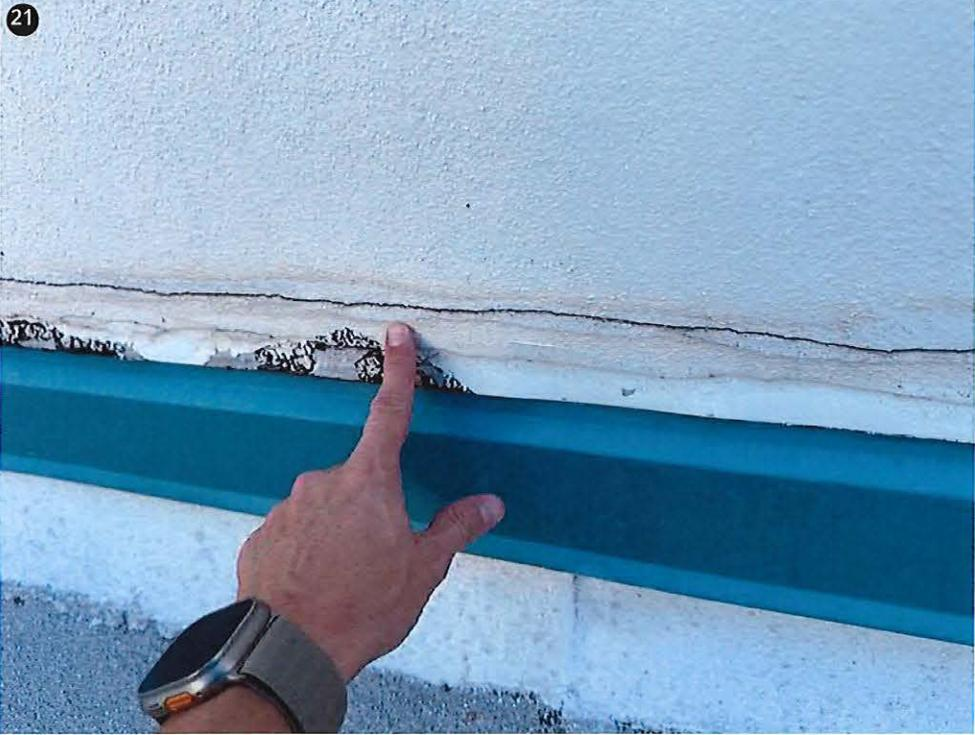
View of large stucco crack forming at the top of the counter flashing, repairs will be needed.
